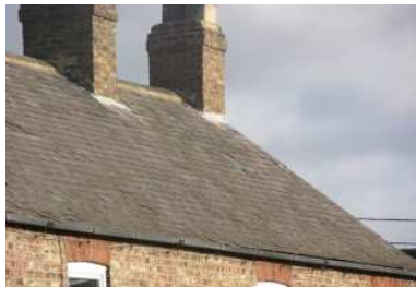
Welsh slate roof
